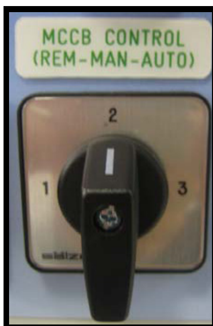
Figure 25. MCCB Control selector switch (-S6)
